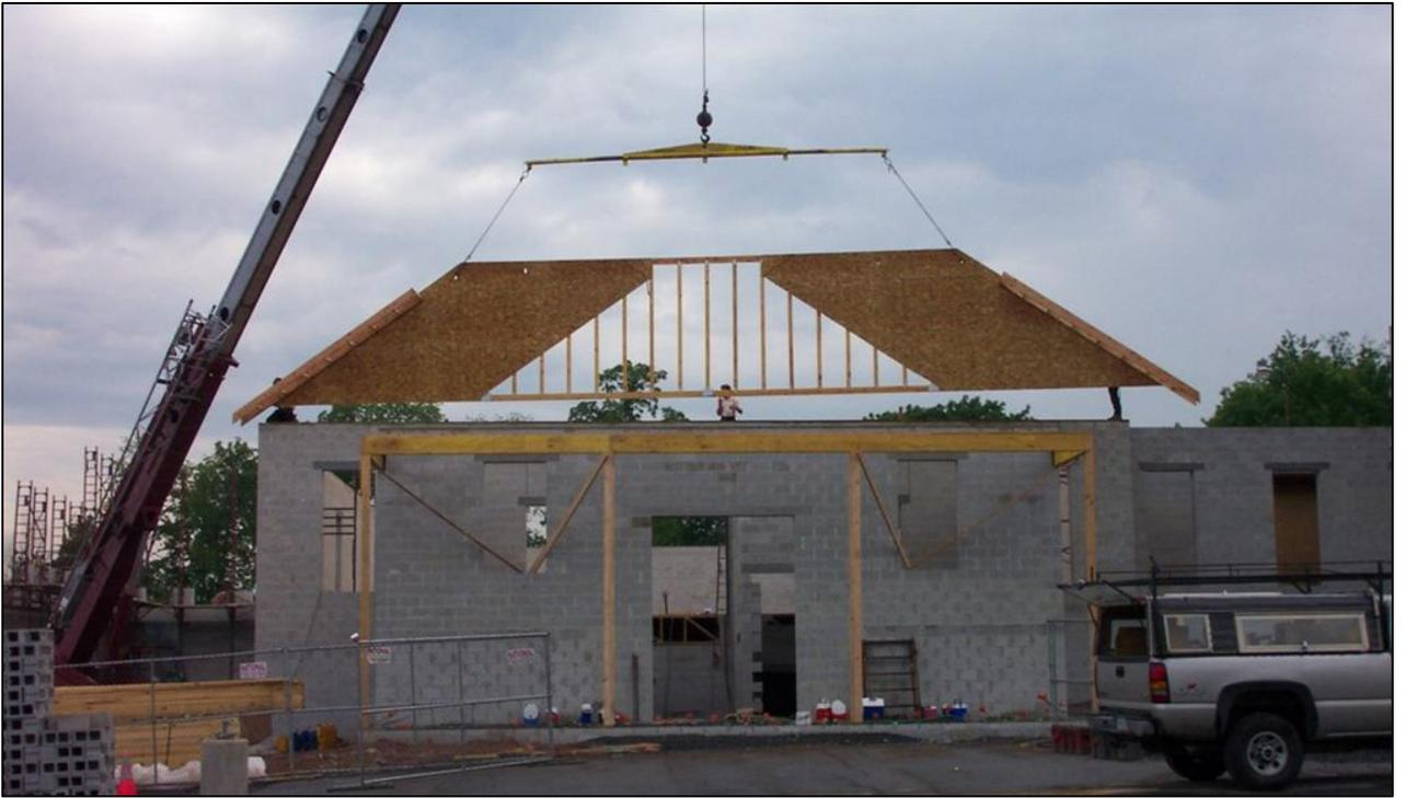
By June of 2005, roof trusses were being put in place by a big crane. 6/16/2005
